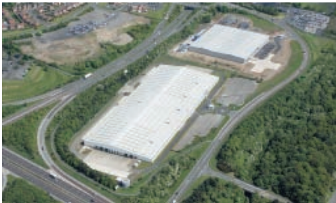
The new Vigo Centre a 250,000sq ft production facility in Washington, UK.
